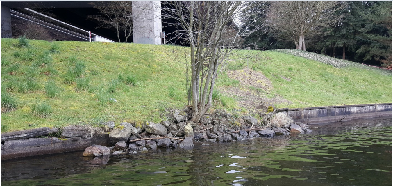
Photo 21. Mercer Island Boat Launch work area taken from the East Channel of Lake Washington. Pipeline alignment will intersect the failing bulkhead at the approximate location of the tree on the shoreline (close up view).
