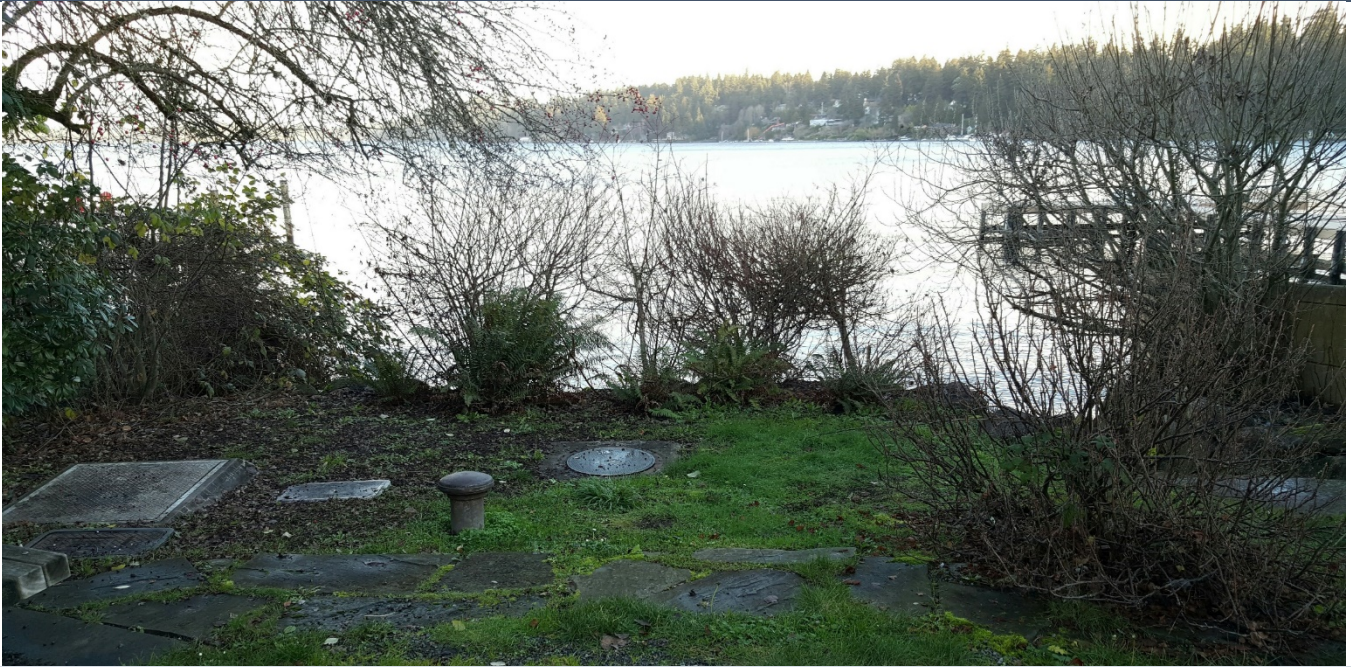
Photo 17. Lift Station 11 adjacent to Lake Washington. Note vault and maintenance hole access; odor control vent.
