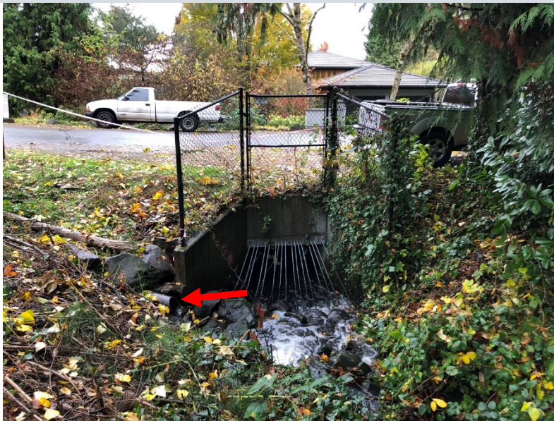
Photo 4. North Mercer Pump Station stream culvert entrance and existing stormwater pipe (red arrow).
