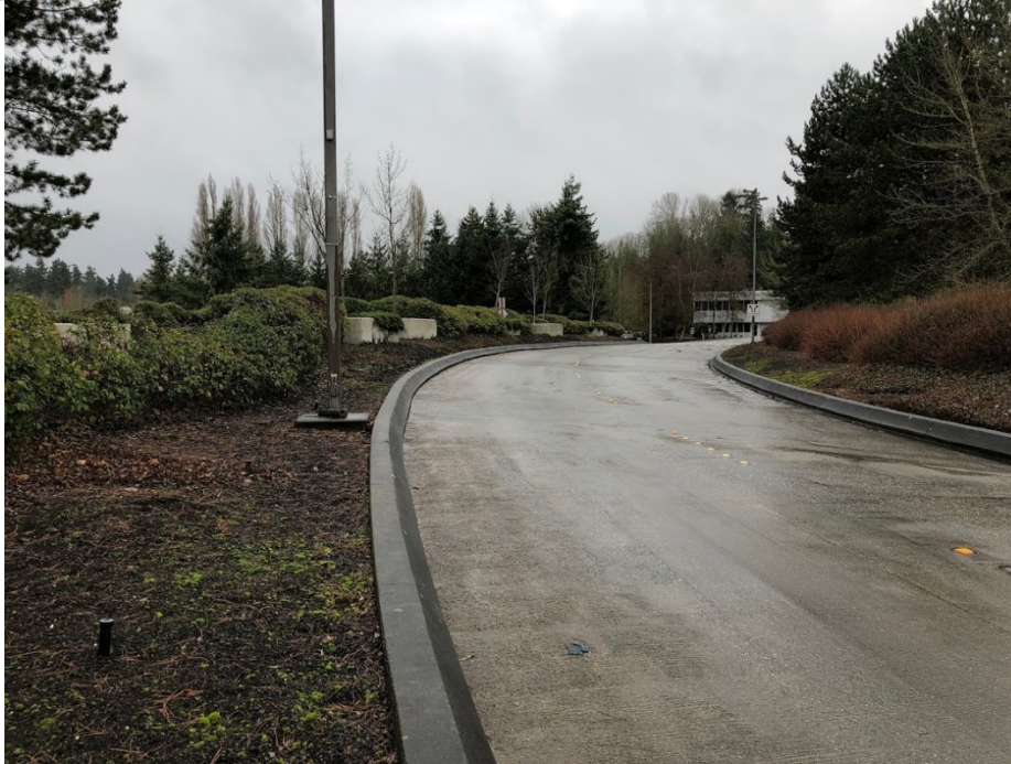
Photo 12. N Mercer Way, looking towards temporary diversion for 96 th Ave Siphon work (9411 SE 33 rd St).
