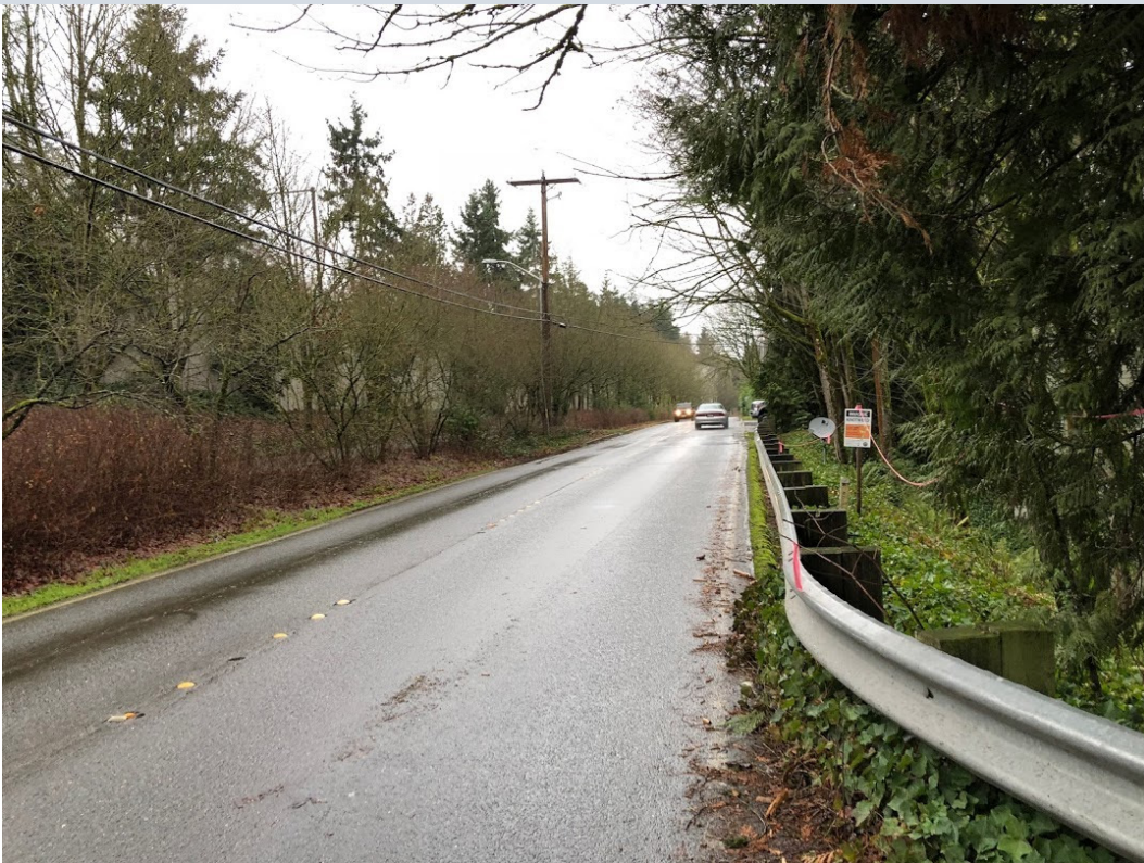
Photo 9. North Mercer Interceptor Route, adjacent to I-90, near piped stream crossing (8446 N Mercer Way).
