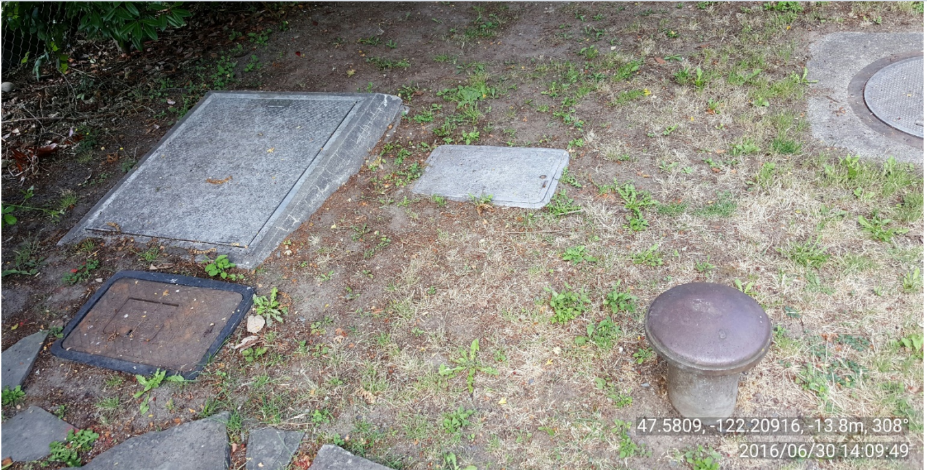
Photo 18. Lift Station 11 existing structures.
